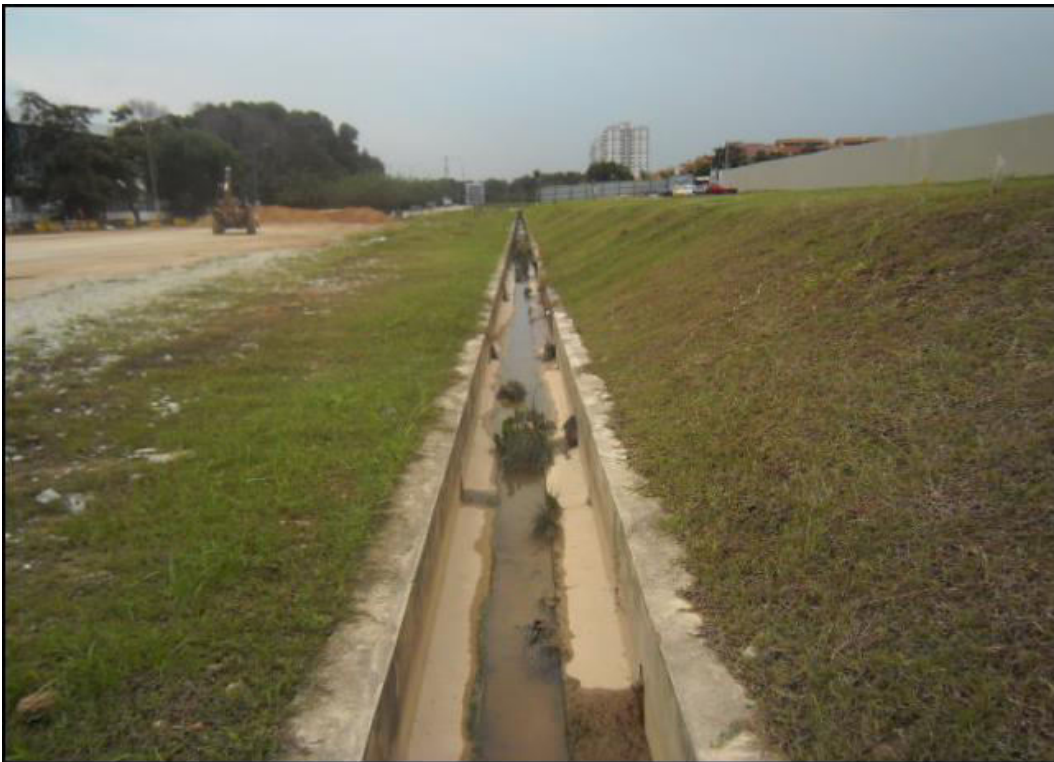
Cemented and cascade drain
