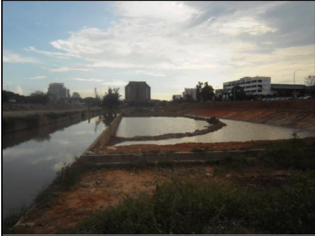
Sediment basins provided next to Sg. Rasau
