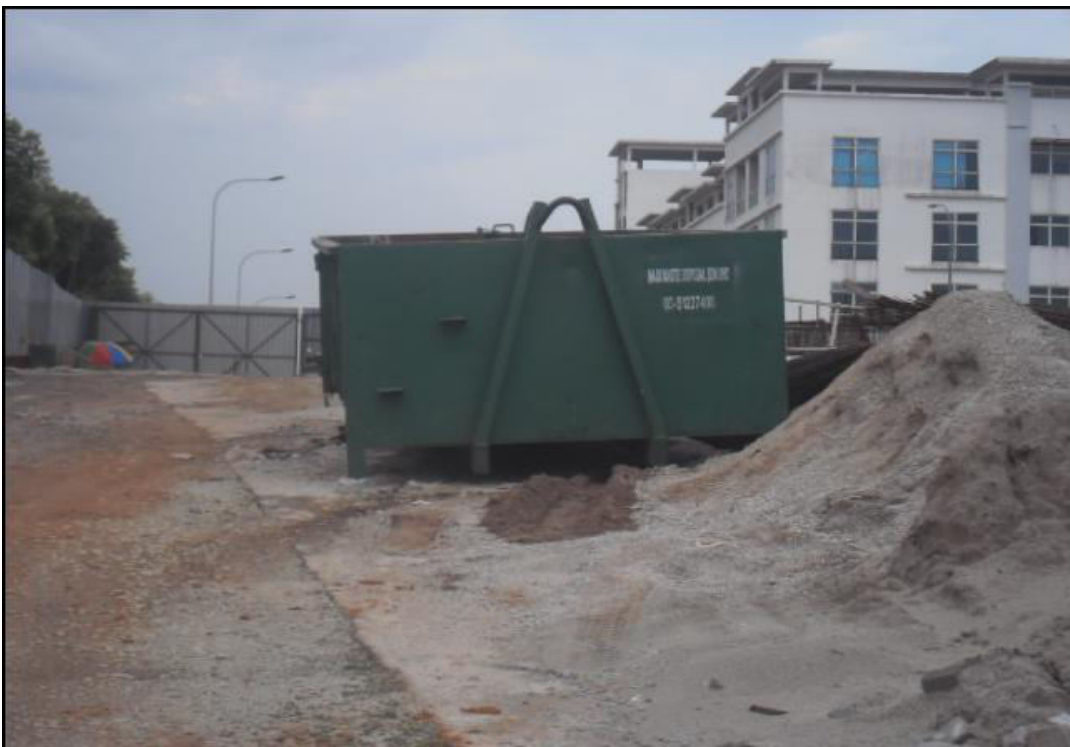
Construction waste stored in proper container and send out from site
