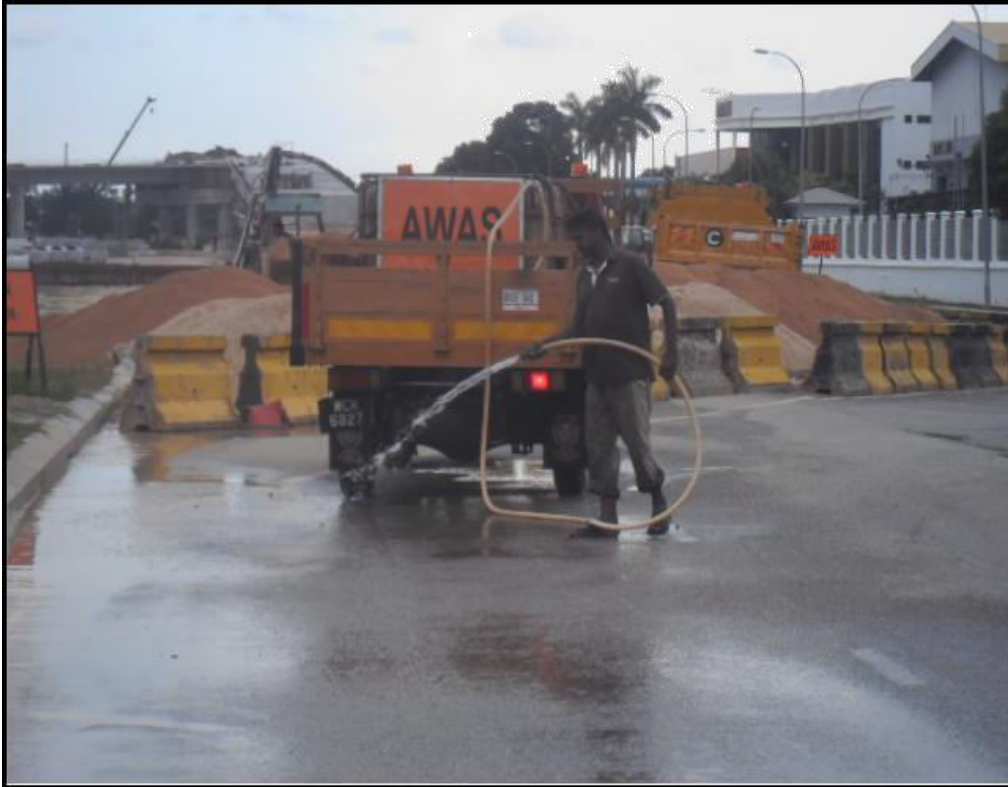
Road watering at truck trails
