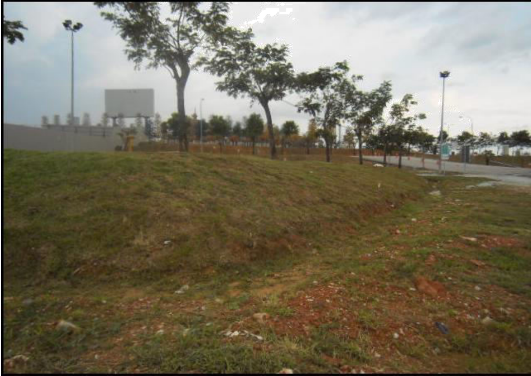
All exposed ground, slopes are turfed
