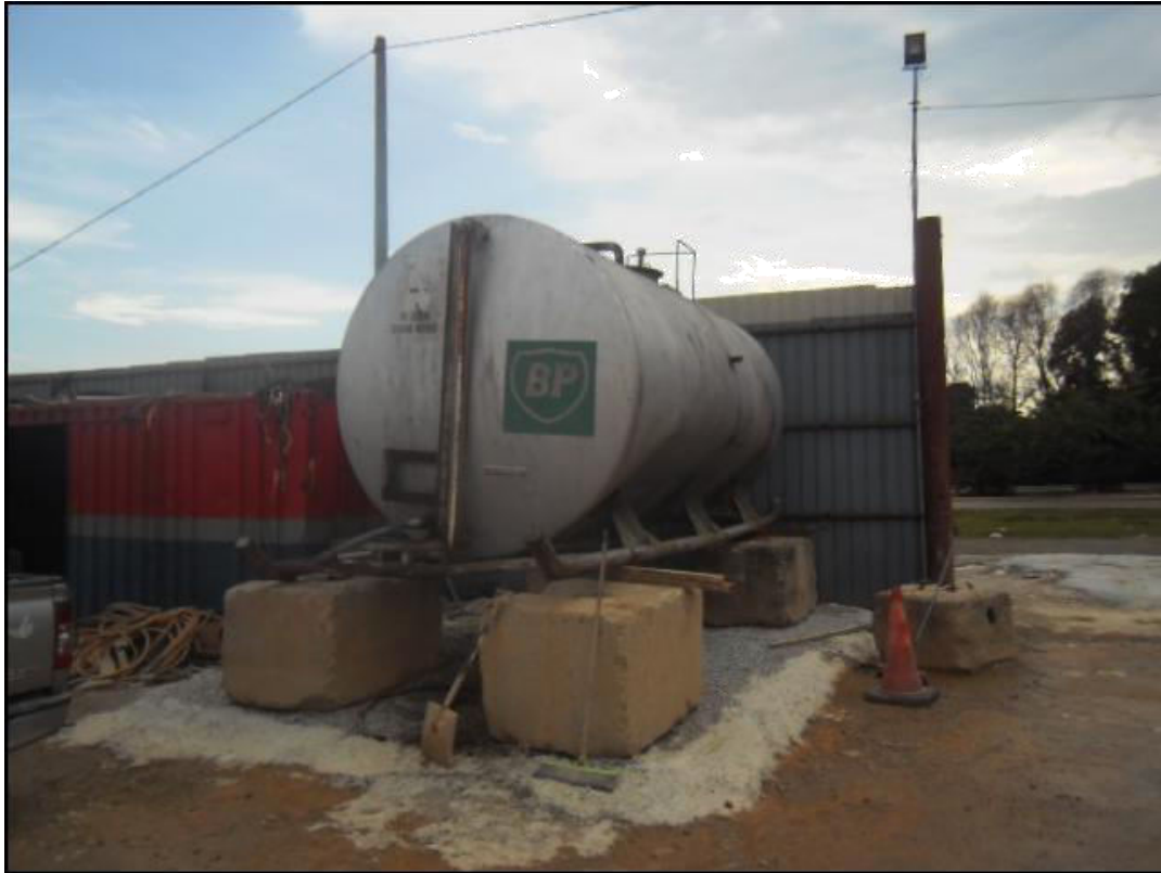
Waste oil contained in demarcated area
