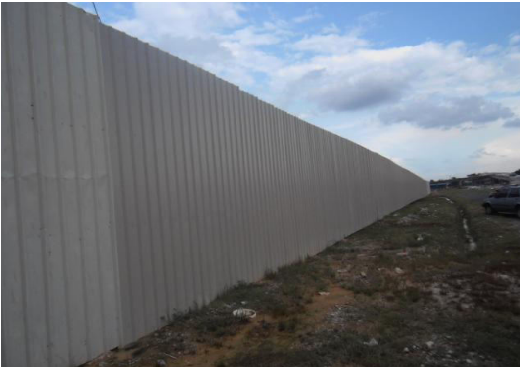
12ft high perimeter fencing provided at site
