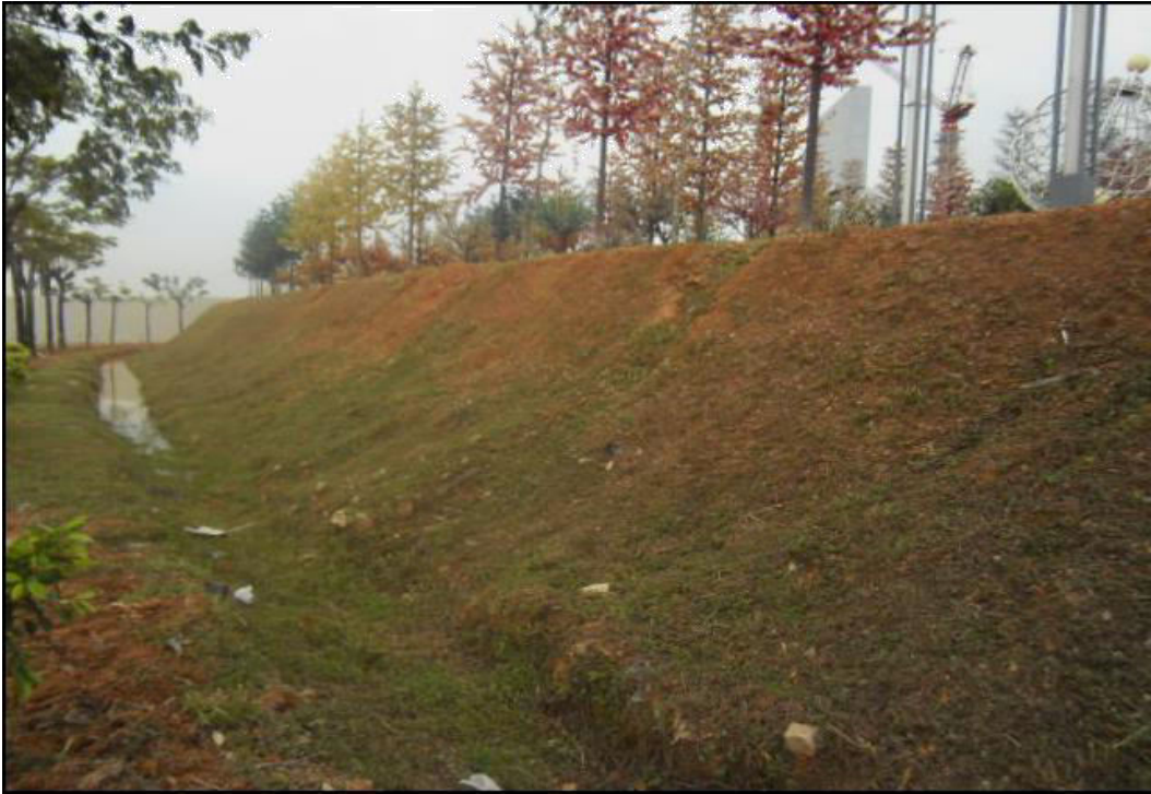
Exposed slope turfed
